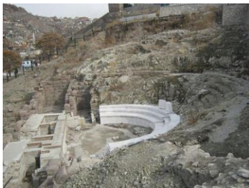
Figure 16. Roman Theater during restoration
