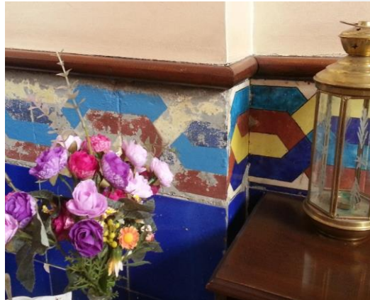
Picture 12, Ankara Gazi Train Station, Inside Wall Maintenance, Özdamar, M., 2015
