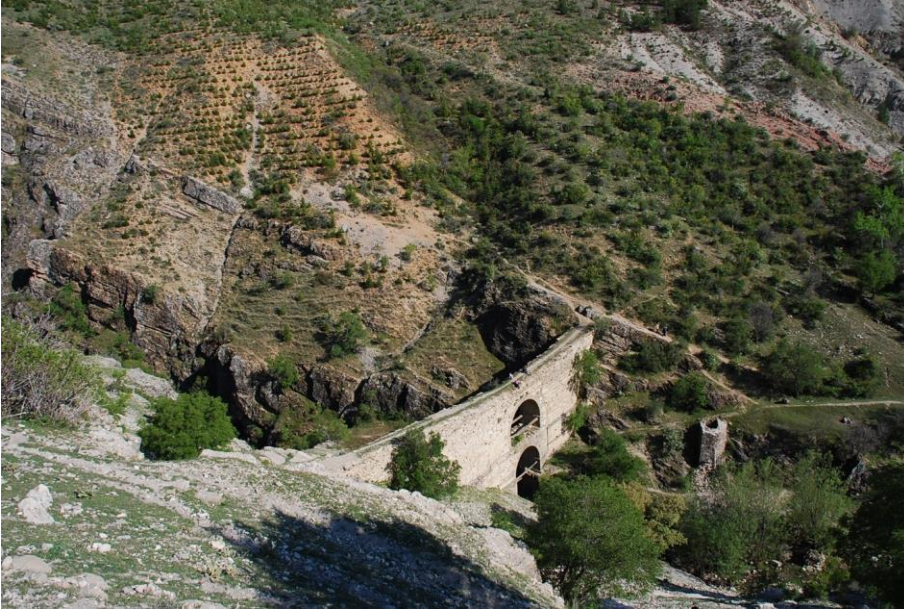
View of Cirimbolu Aqueduct
